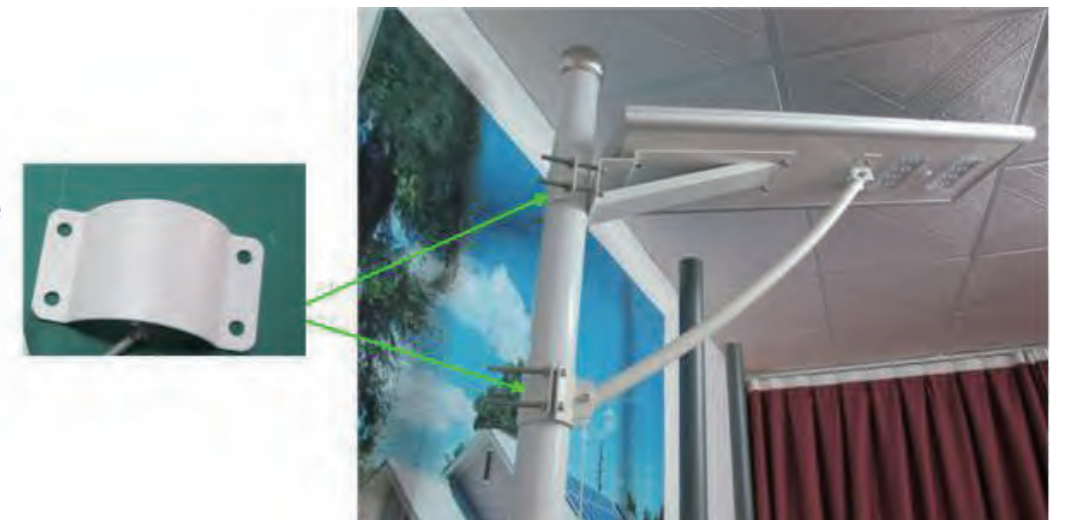
Step 6: Mount the light fixture/box on the pole.
